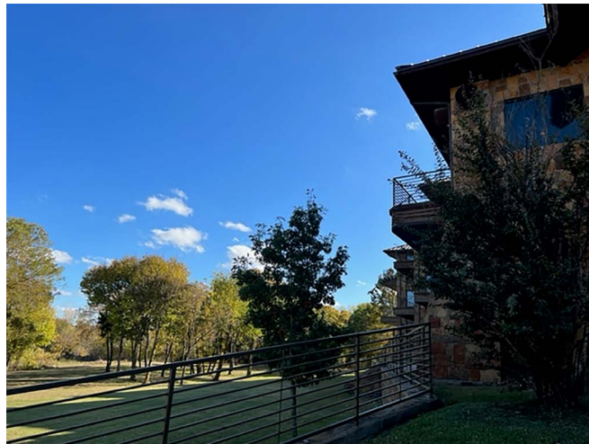
NORTHEAST EDGE OF BUILDING FACING SOUTH
